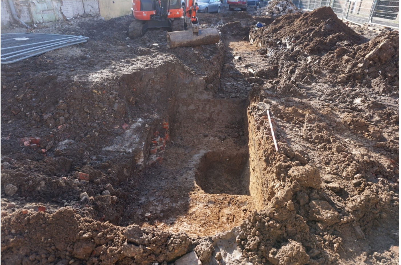
Plate 4: Looking SW at trench 1
