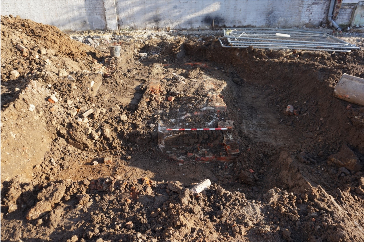
Plate 8: Looking SE at brick built mechanic pit (109) exposed in trench D2. Pitt was filled in with cast concrete. Tank is buried under heras fencing panels.
