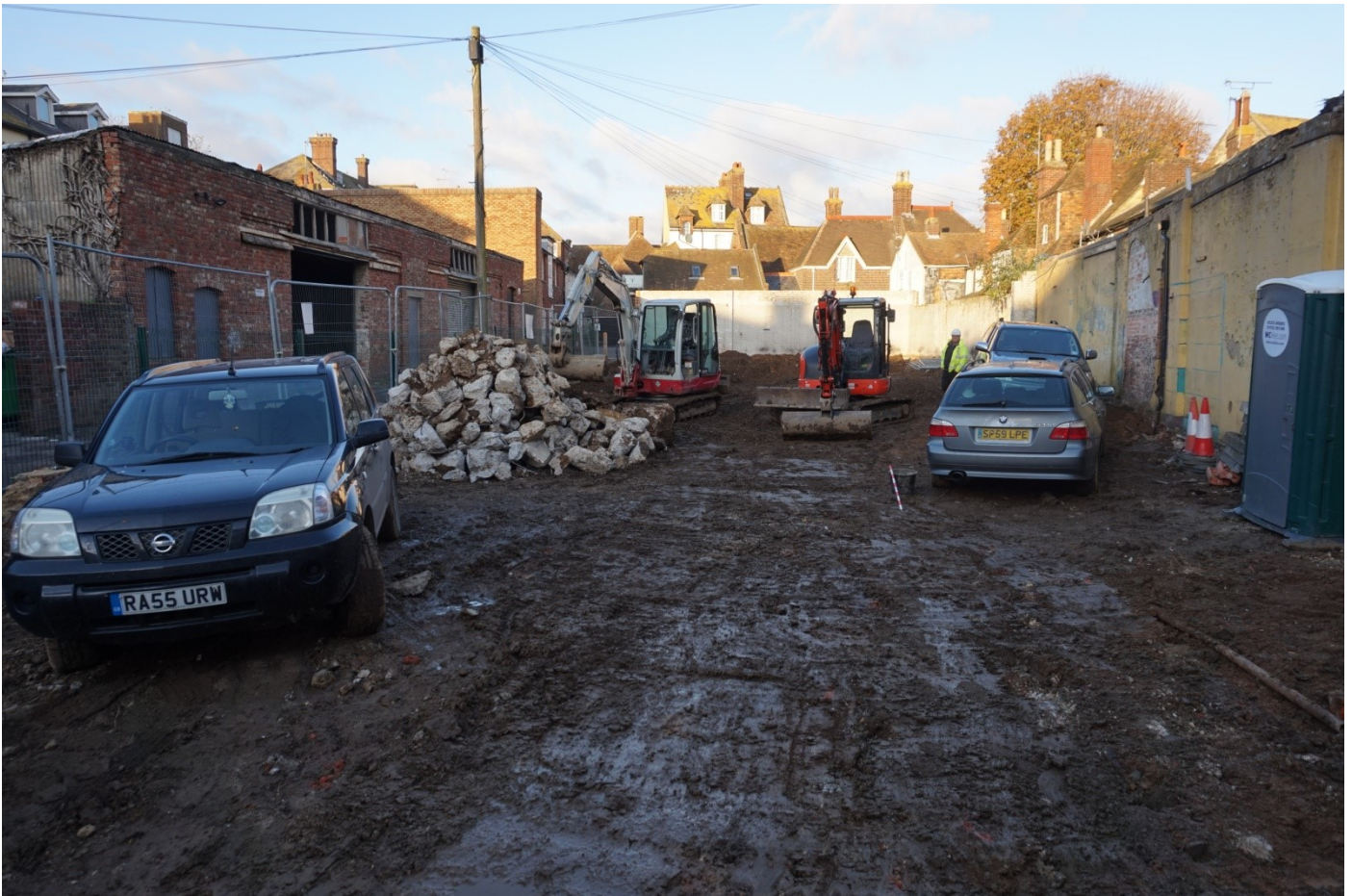
Plate 1: Looking NNE at the site. Pile of concrete came from demolition of mechanic pit.
