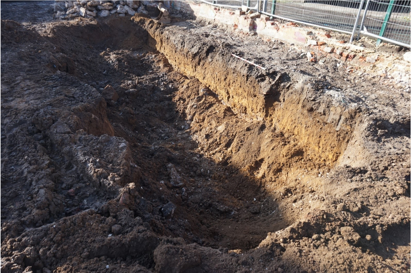
Plate 6: Trench D1 excavated in order to remove concrete mechanic pit – recorded as trench 2
